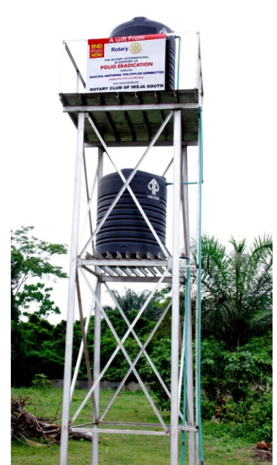
Rotary Motorized borehole at African Church School, Igbore, Obafemi Owode LGA, Ogun state
