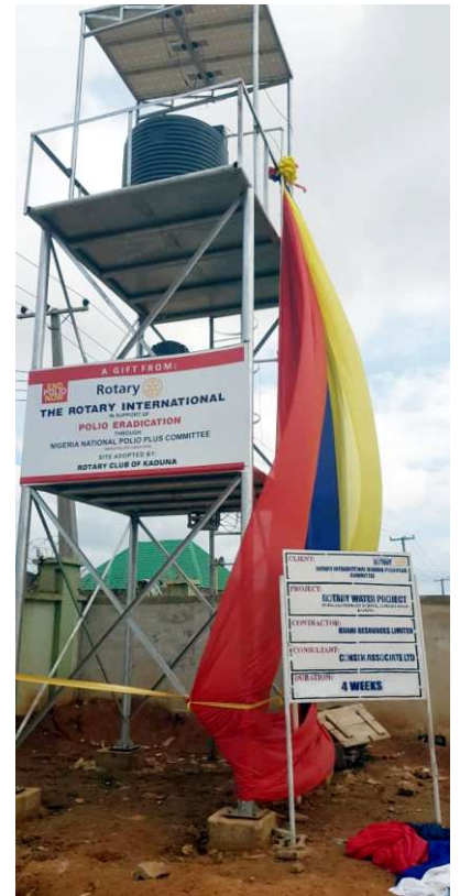
Rotary Solar Borehole in LEA Primary School, Kaduna
